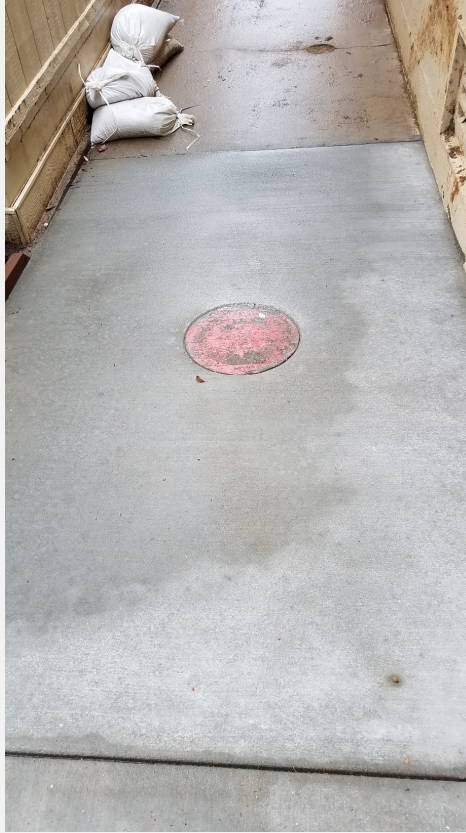
MHS: Water valve replacement
